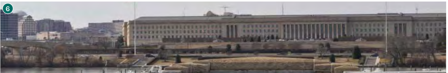
View of the Pentagon Building from Humpback Bridge
