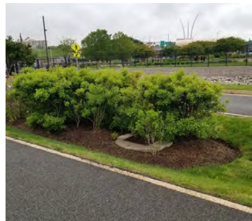
Corridor 5 VACP Existing Bioretention Area
