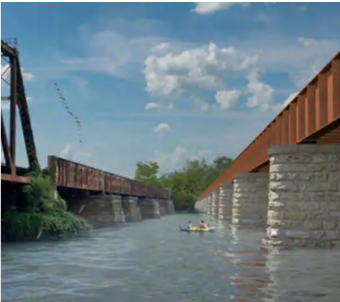
Long Bridge Rail Pedestrian/Bike Bridge
