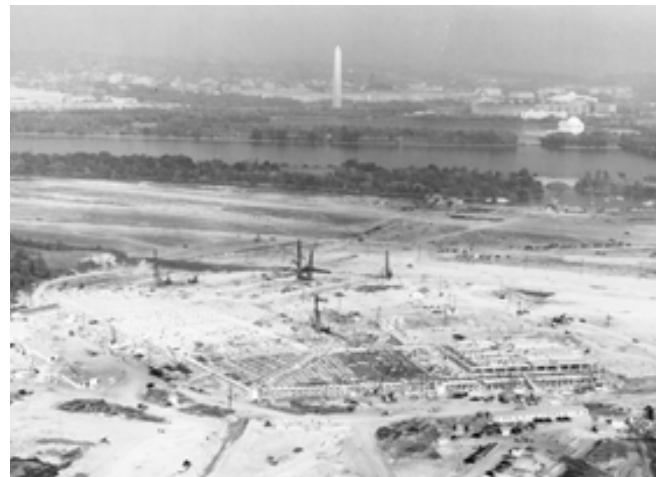
Construction on the First Side of the Pentagon, November 5, 1941
