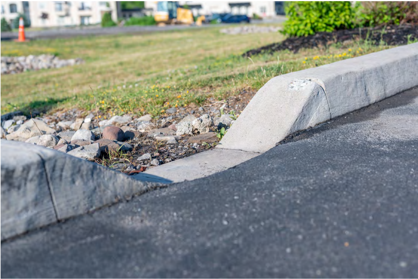
Swales Used to Transport Stormwater Runoff
