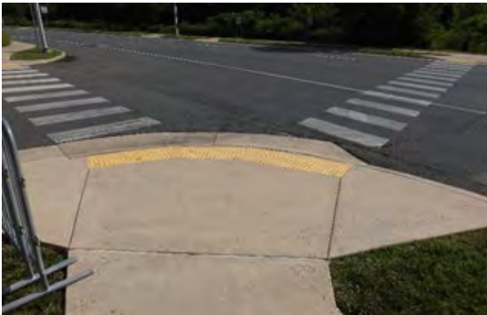
Realign Sidewalk Ramp/Pedestrian Crossing
