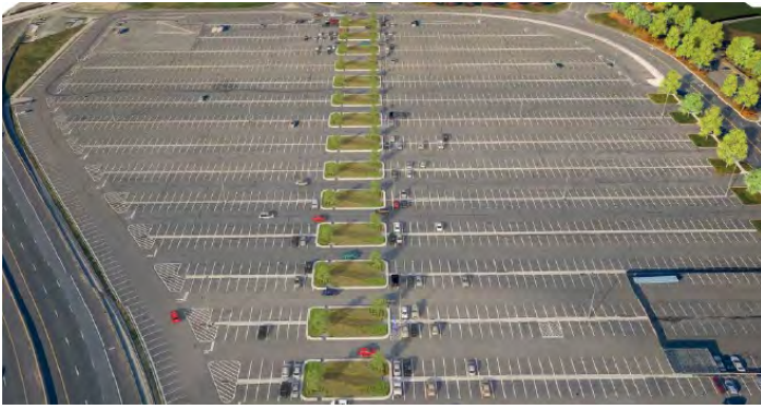
North Parking Bioretention
