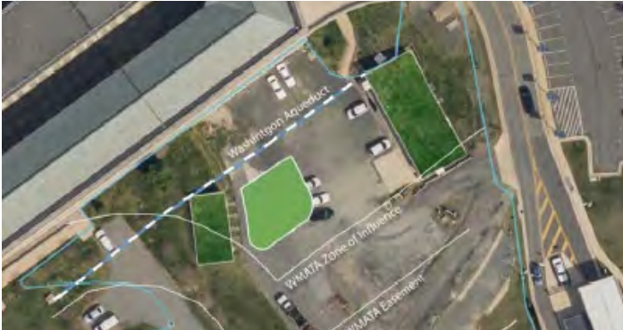
Old East Loading Dock
