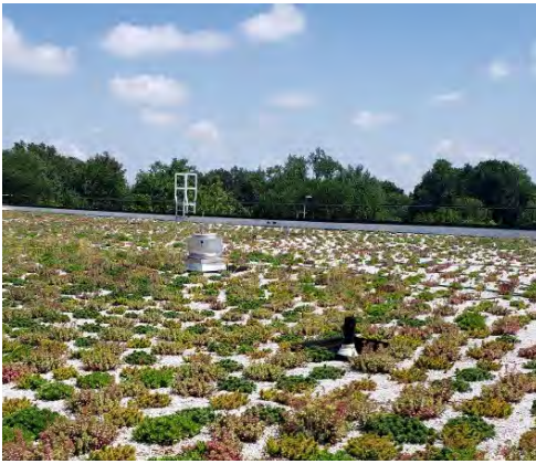
PSOC Vegetated Roof
