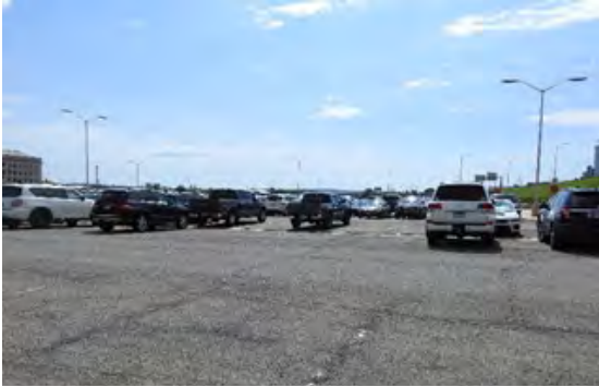
Rehabilitate Deteriorated Pavement in South Parking Lot
