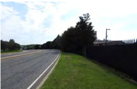
Install Missing Sidewalk Section
