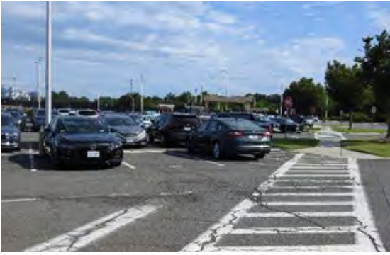
Rehabilitate Deteriorated Pavement in North Parking Lot
