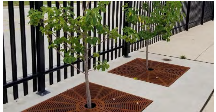
Current Tree Box Filter in Slug Lane, Southeast Parking
