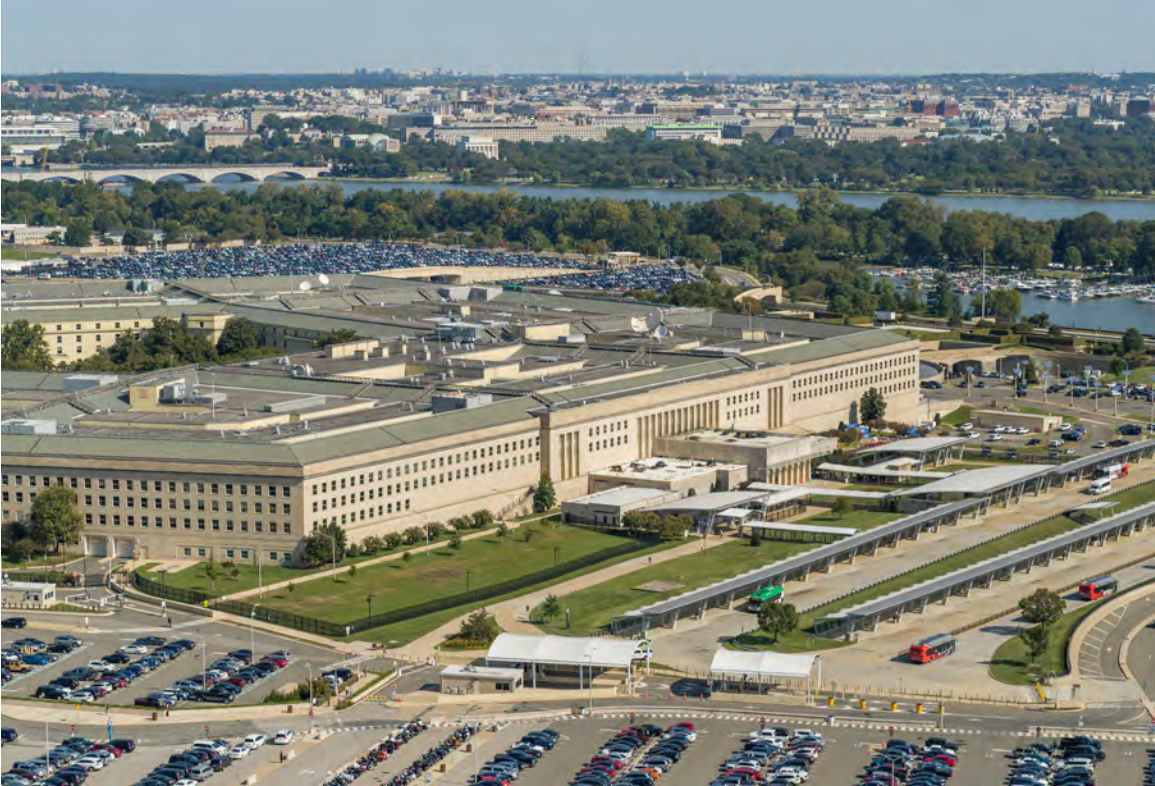
Aerial View of the Pentagon Transit Center
